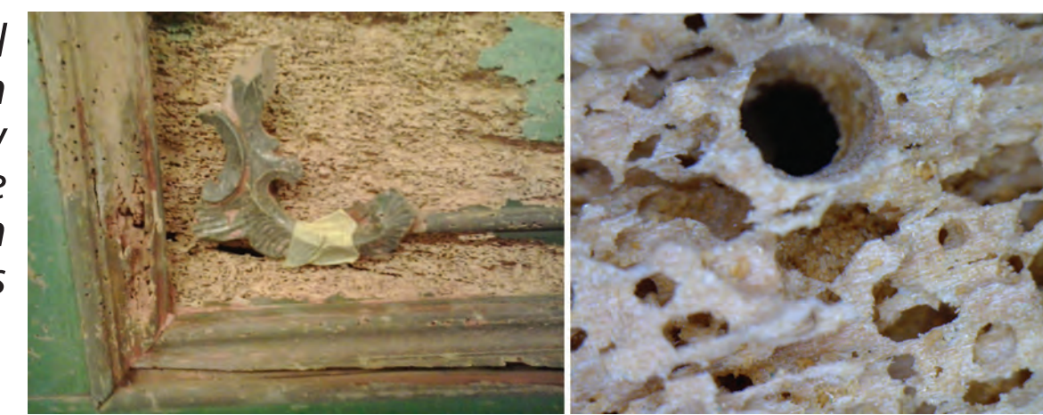
Part of the wall panel before restoration damaged by woodworms, and the macro photo with woodworm caverns
