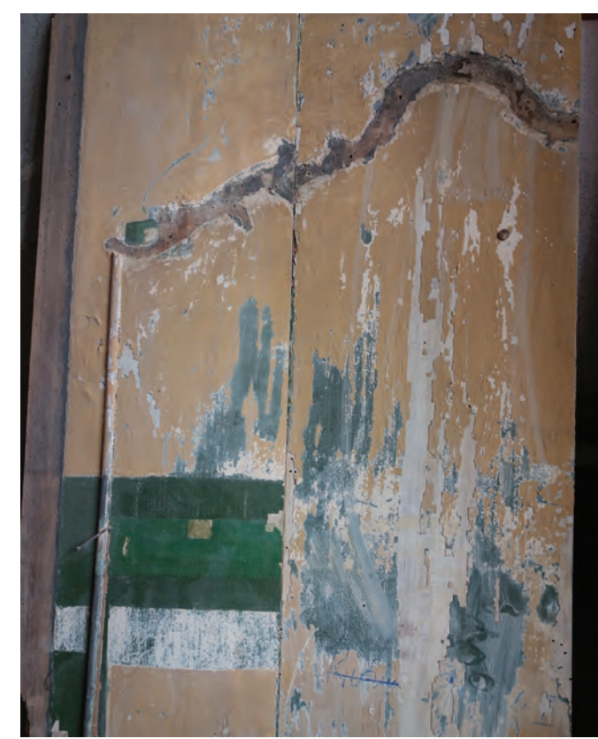
Wood wall panels before restoration. Over-coating removal tests on the wood panels.
