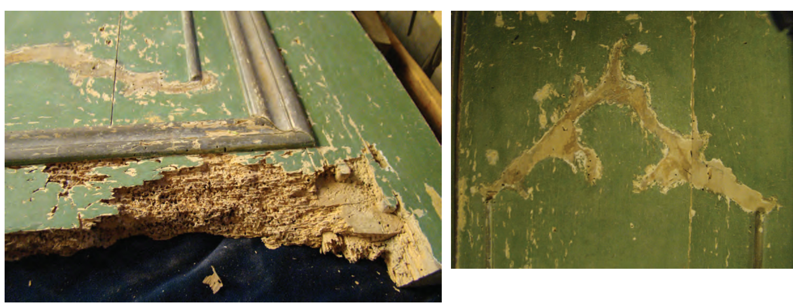
Wood wall panels before restoration. Over-coating removal tests on the wood panels.
