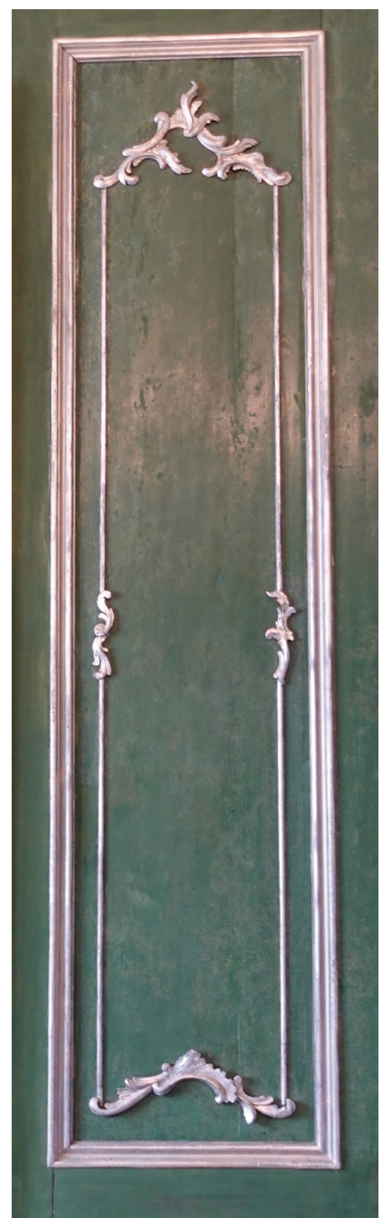
The wall panel after restoration.
