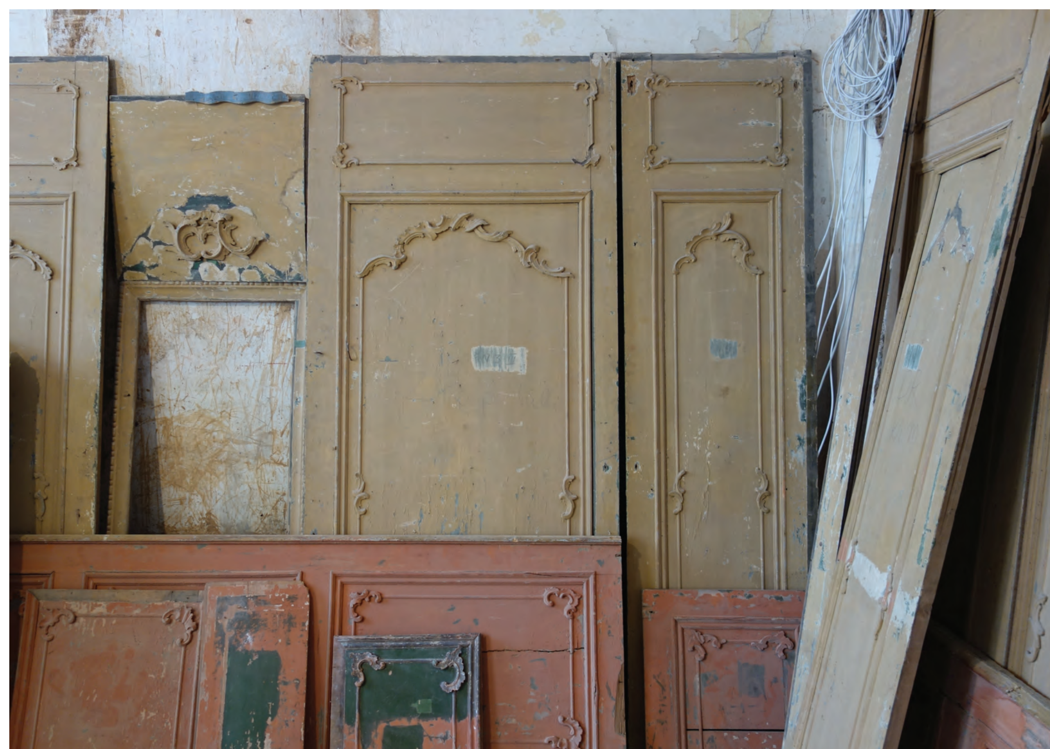
Wood wall panels before restoration. Over-coating removal tests on the wood panels.
