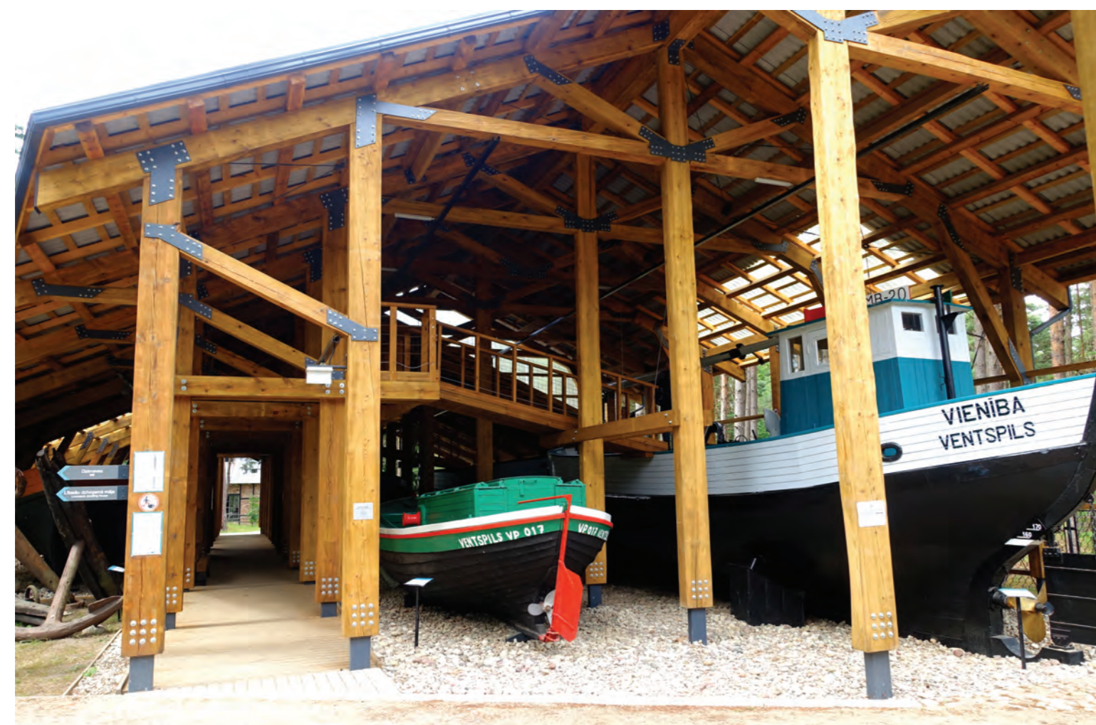
Fig. 3, 4 The new Boat House building of the Seaside Open-Air Museum
