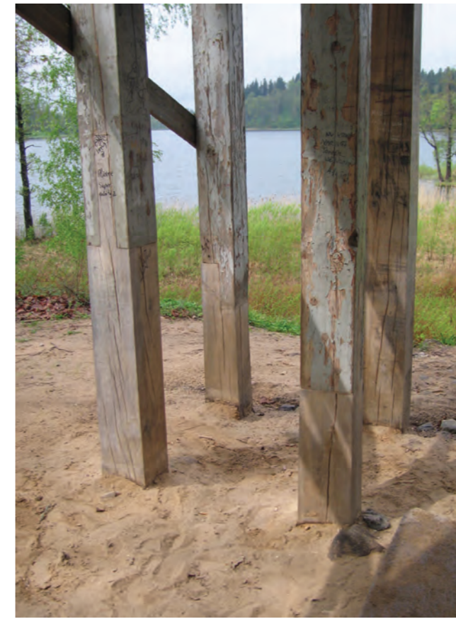
Oak end pieces added to pillars, 2002
