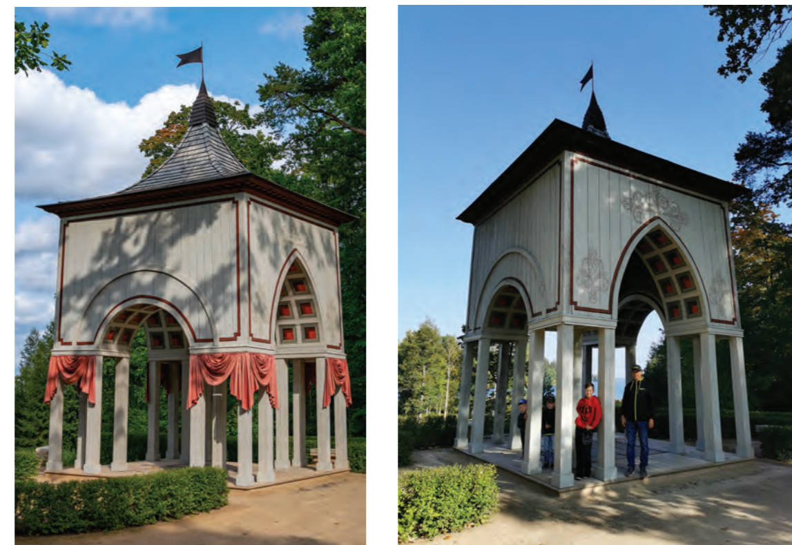
The drapery fabric should be matte, with a finished edge, with little creasing (empire style) and its length should be proportional to the length of the pillar
