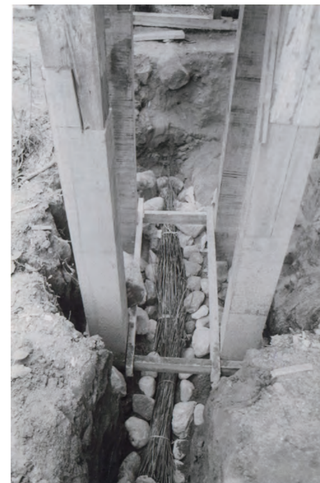
Fascines are placed to allow water flow to the lake
