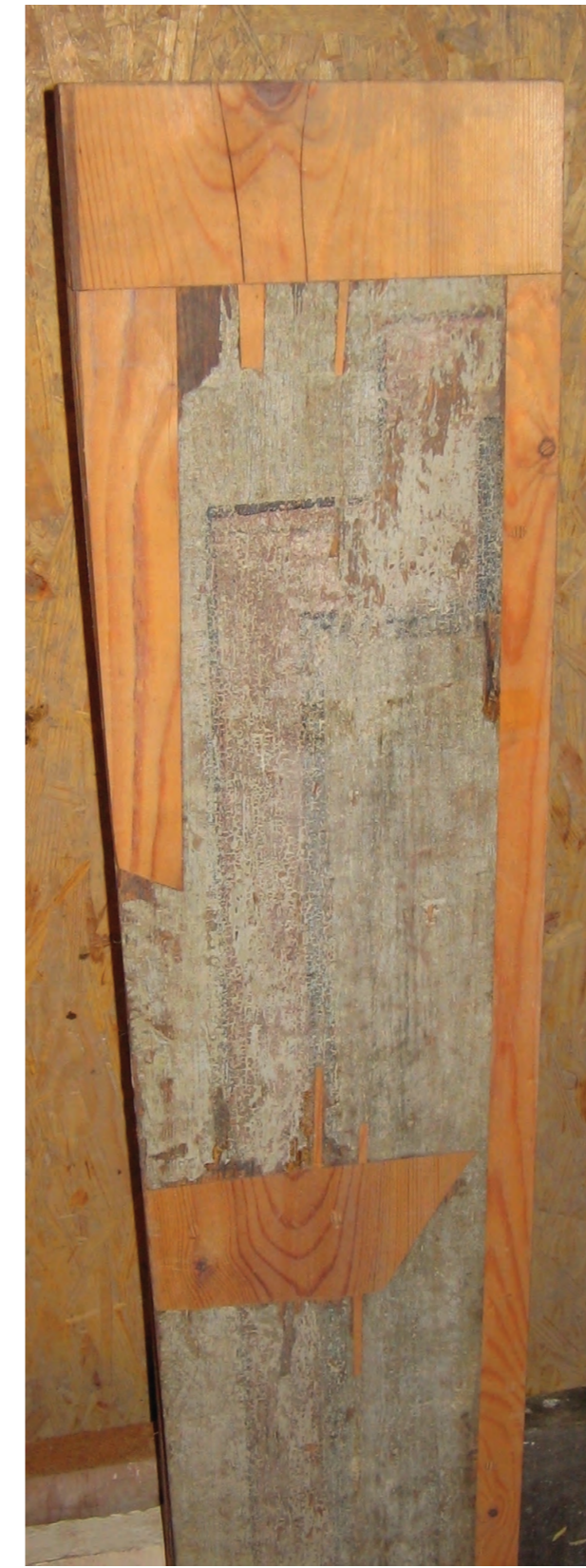
Board from the facade, prosthesis done on site
