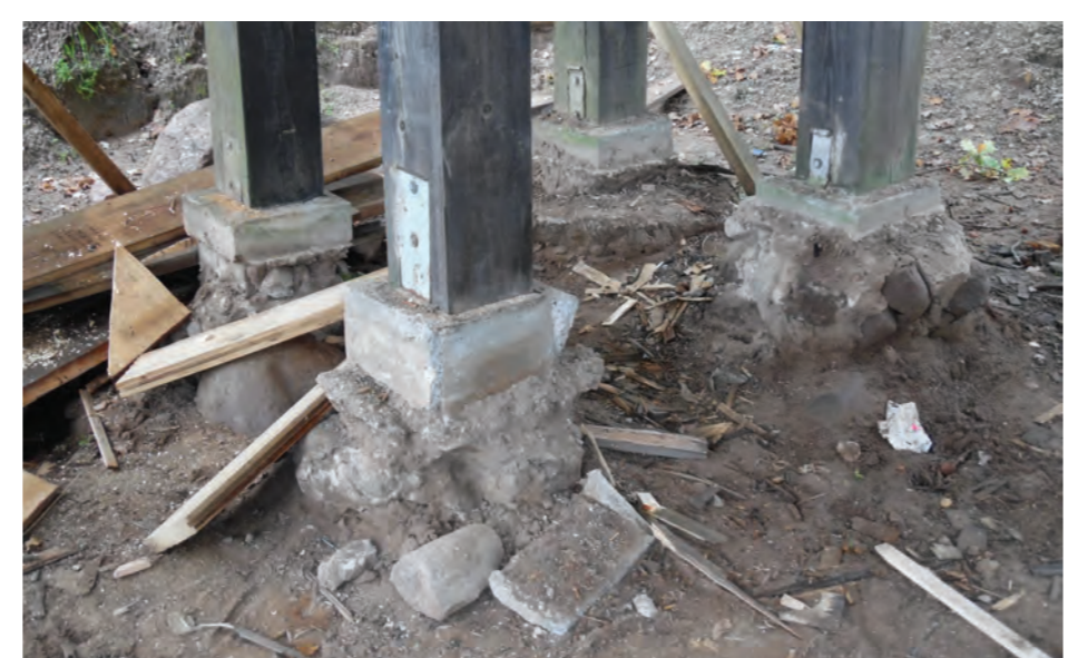
In 2017 oak end pieces are shortened. These pillars were installed in the first decade of the 21st century. Also in 2017, the foundation is concreted according to the 1956 model. In 1956 salvage work was performed but in 2017 the funding was given for "restoration"
