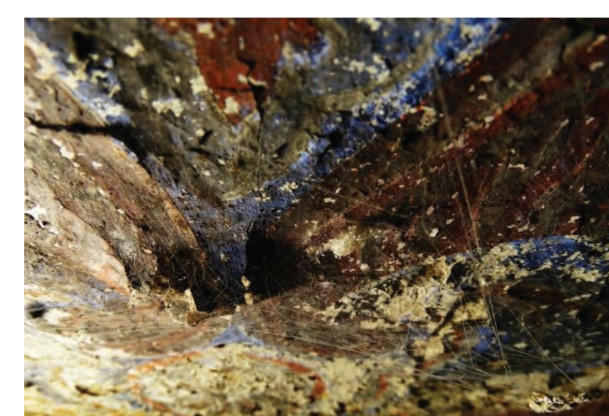
Fig. 4. Biological damage to the VII ornament of the monumentally decorative ceiling painting composition of the 1st floor of the Valmiermuiža palace tower
