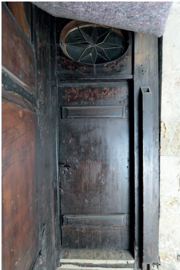
Image 4. A coloured relief can be discerned in the brown paint and the painting of decorative ornaments under the brown paint.
