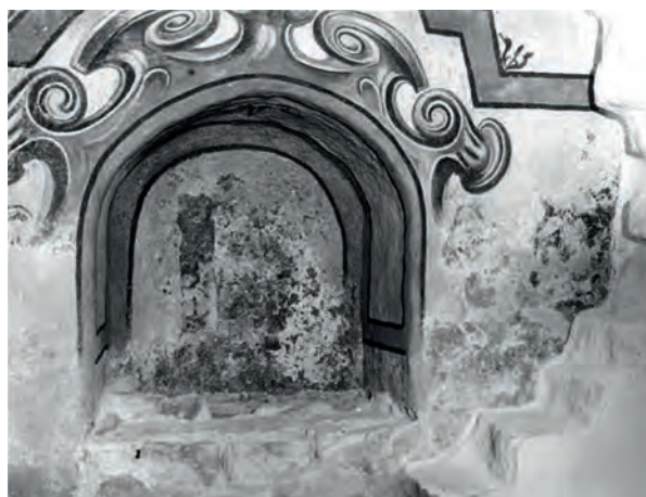
Image 1. Restoration of fireplace decoration, 20 th century, 90s. Rīga, Skārnu street 2
