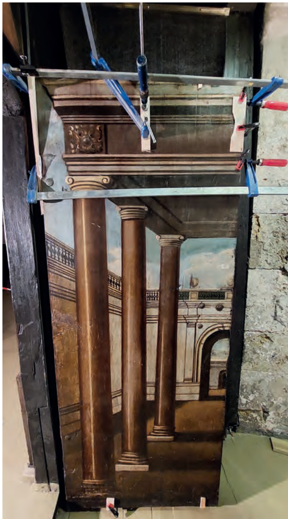
Image 7. Gluing process of the cracks and the wooden inserts in the door with glue clamps, photo Aigars Pilenieks
