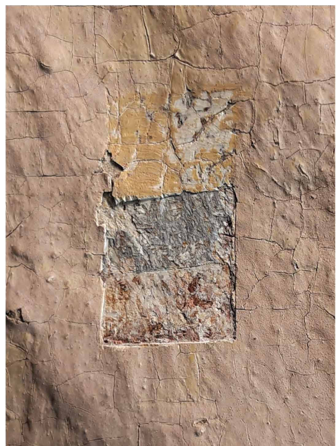
Fig. 3. Exposed sounding area. Photo: Sarmīte Balode
