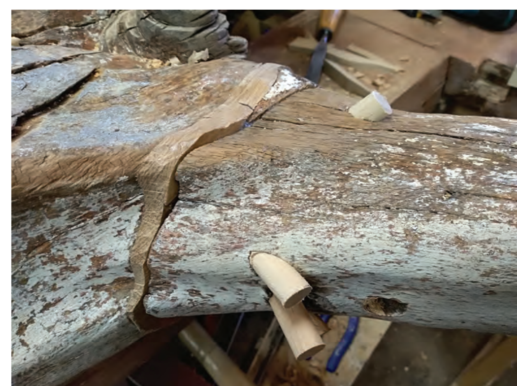
Fig. 10. Additional strengthening of hands with pins. Photo: Aigars Pilenieks
