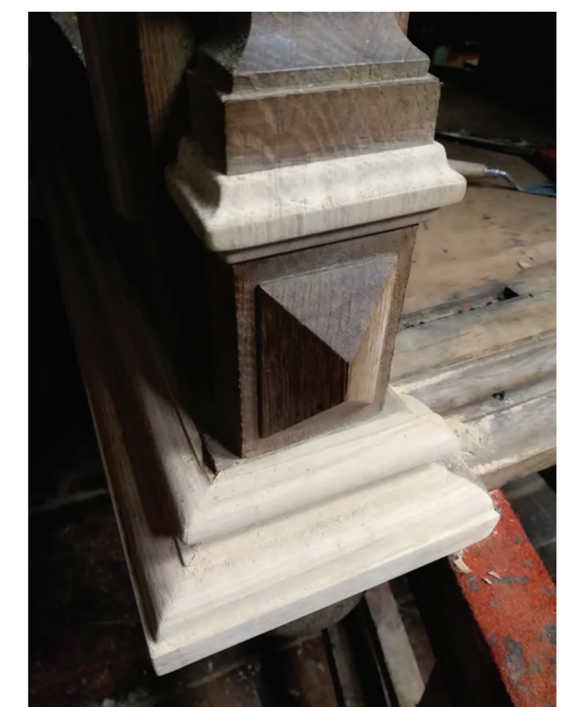
Fig. 8. New profile strips have been incorporated. Photo: Aigars Pilenieks
